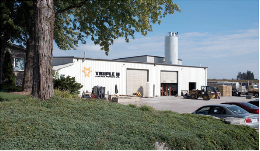
Home of Triple H Concrete Products
