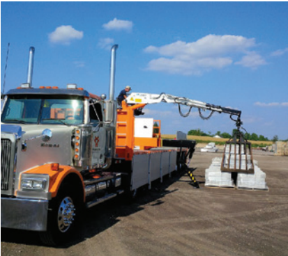
Loading pavers for shipping
